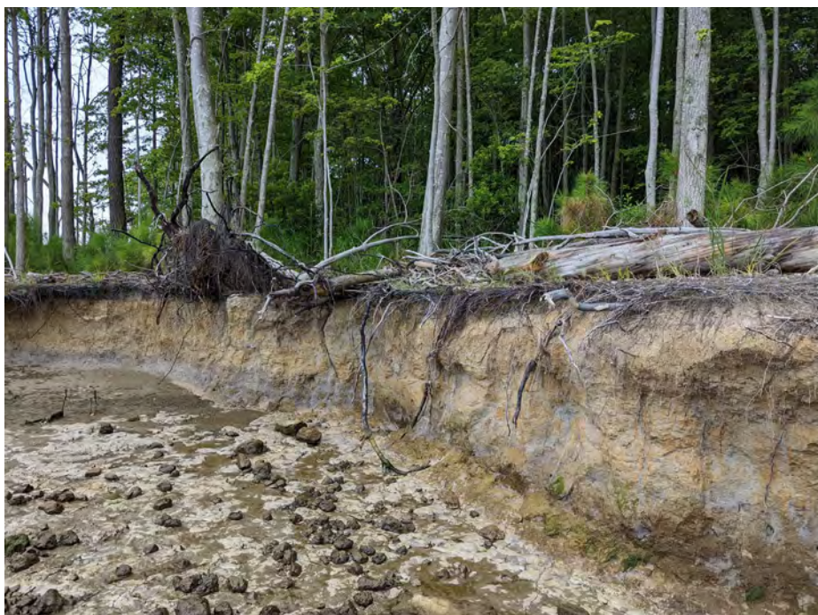
Erosion at Franklin Point, pre-restoration (2022). PHOTO, ARUNDEL RIVERS FEDERATION
